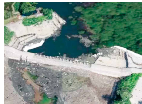
[Figure 5] Yuda Check Dam point cloud data
